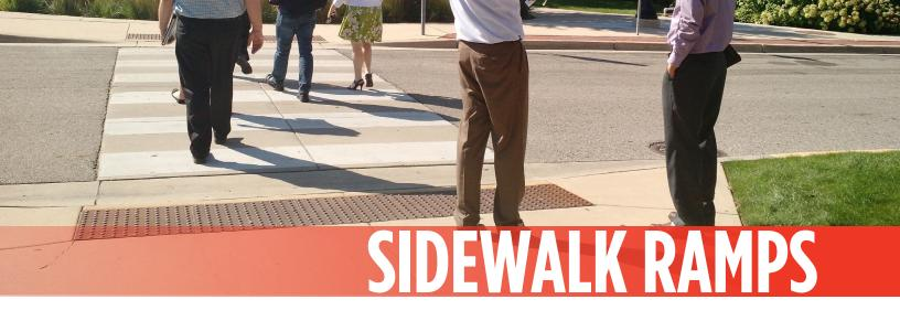
Sidewalk ramps are short ramps cutting through a curb or built up to it that provide the transition from the sidewalk to the street. Sidewalk ramps are essential in providing mobility to persons with mobility impairments. They also contribute to overall utility and livability for a wide range of users, including people pushing strollers, delivery carts, or dollies; people pulling luggage or utility carts; and people walking with a cane, crutches or a bicycle.
